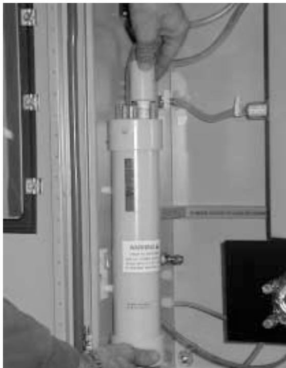
*Figure 5-9: Removing the UV Reactor Assembly*
